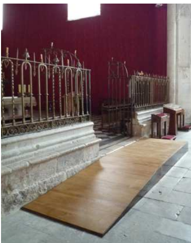
Ramp for access to the altar.
