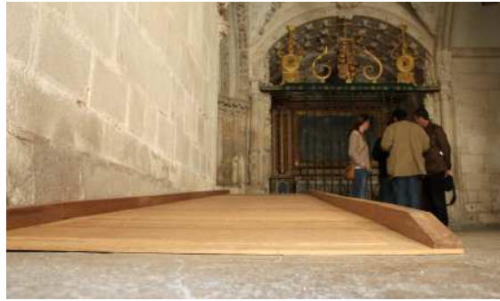
Non-slip ramp with lateral protection.
