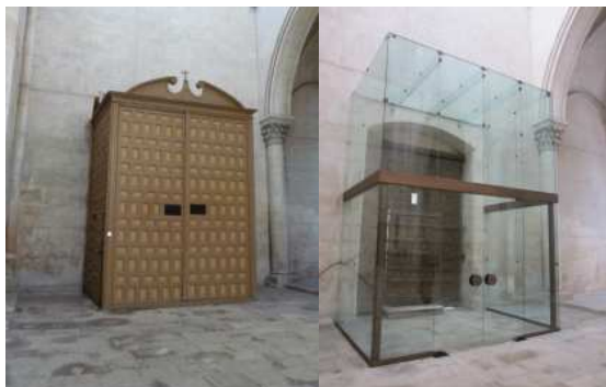
Before and after replacing the wooden porch with a glass windbreak at Las Huelgas Monastery.
