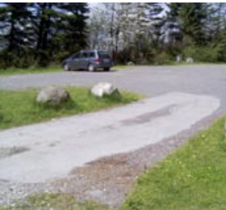
An example of how well hidden an inductive sensor is: only the lines where the cables have been buried in the ground are noticeable. Photo from Store Dyrehave in Denmark, where inductive sensors have been in continuous use since 1977.
